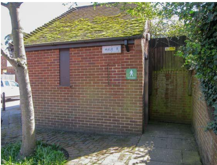
Signage on male toilets
