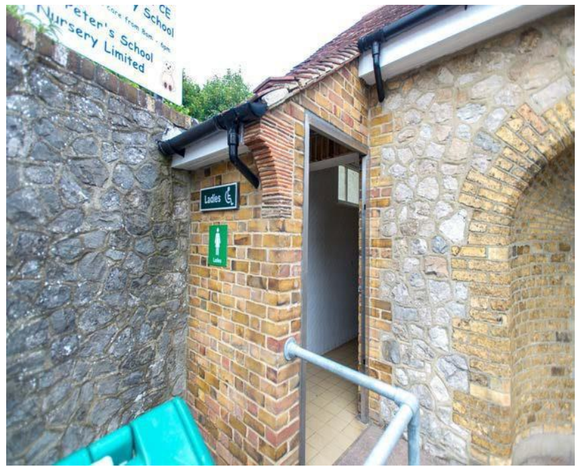
Female toilet entrance
