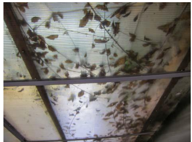
Roof light panels Wrotham Toilets
